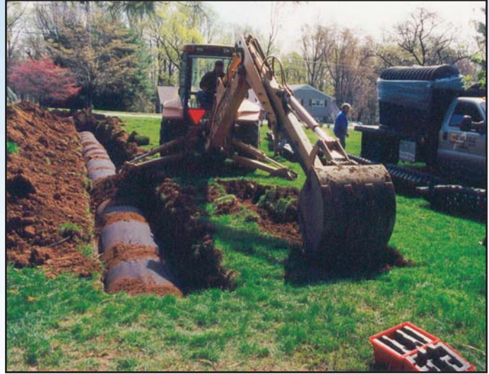
Trench installation demonstrating minimal disturbance of land.
